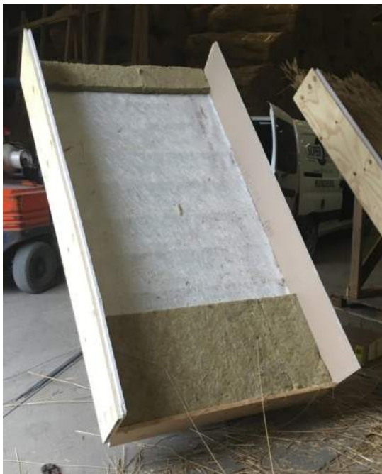
Photo 3: Laying of Sepatec and edge insulation on batten layers (roof models 2 and 3).
